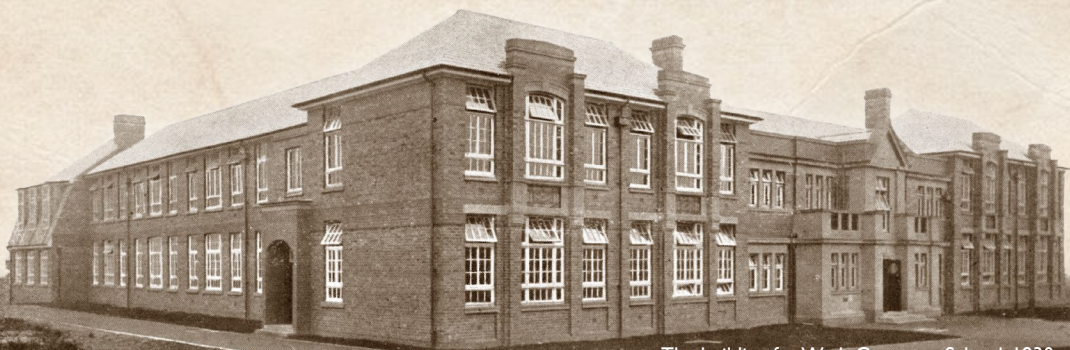
The building for Wath Grammar School, 1930
